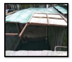
For the partial sedimentation, wastewater from all sewage lines fall into a large septic tank (Fig:5) (20x25x22 feet) which is constructed in the parking area of university. After partial sedimentation, wastewater from university enters into the main sewage drain in Shadman, Lahore and further moves to main wastewater treatment plant of city that is located at 22km away from university in Gulshan-eravi. Lahore
